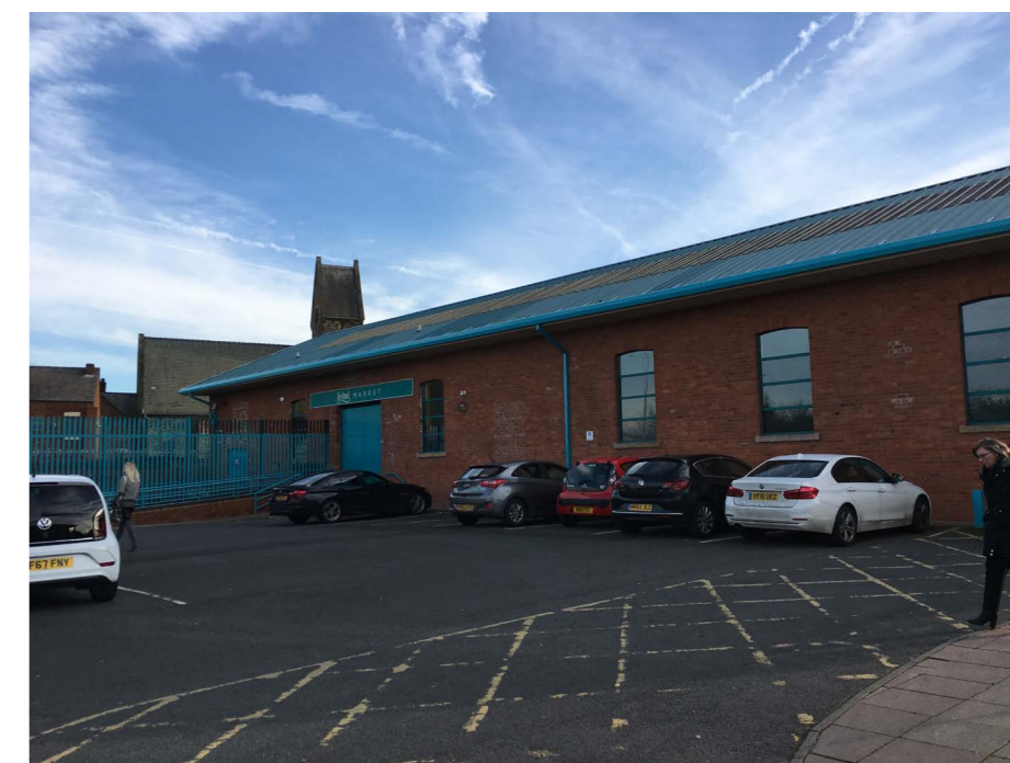
Leyland Market Hall and Car park
